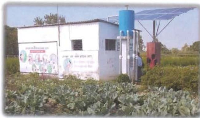
Community Based Solar Power Irrigation
